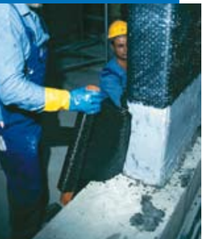
Application de Mapewrap C Uni-Ax
